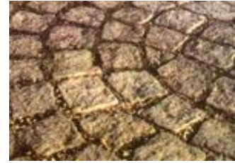
'Rough Punched' - roughly hewn with high spots chiselled off.
