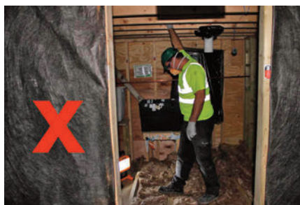
...or to walk on the joists like this
