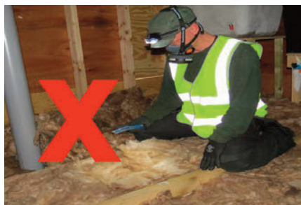
It is not safe to either crawl on the joists parallel with them like this
