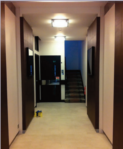
Internal repairs and redecorations to a prestigious West End residential block
