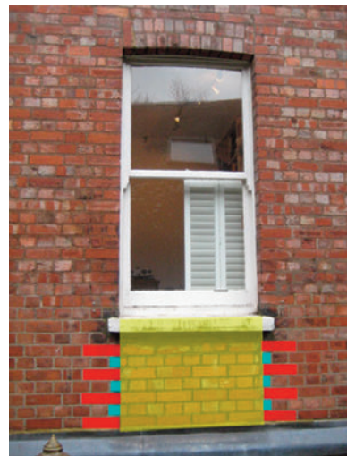
Structural alterations to a West London block in a conservation area
