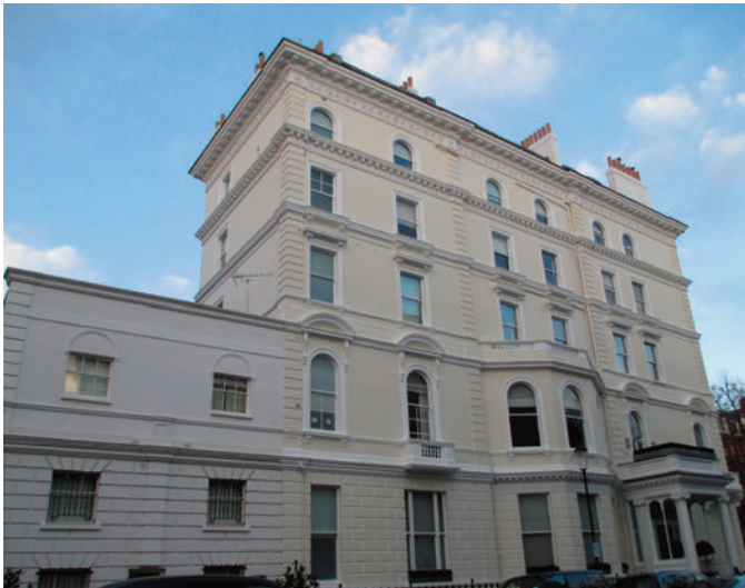
Repairs and restoration to Grade II listed central London residence
