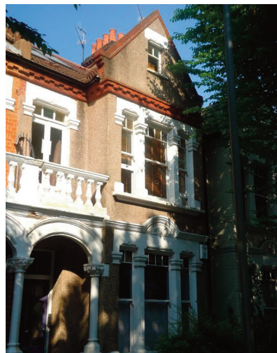
Building survey of a Victorian terrace house for a residential private client.
