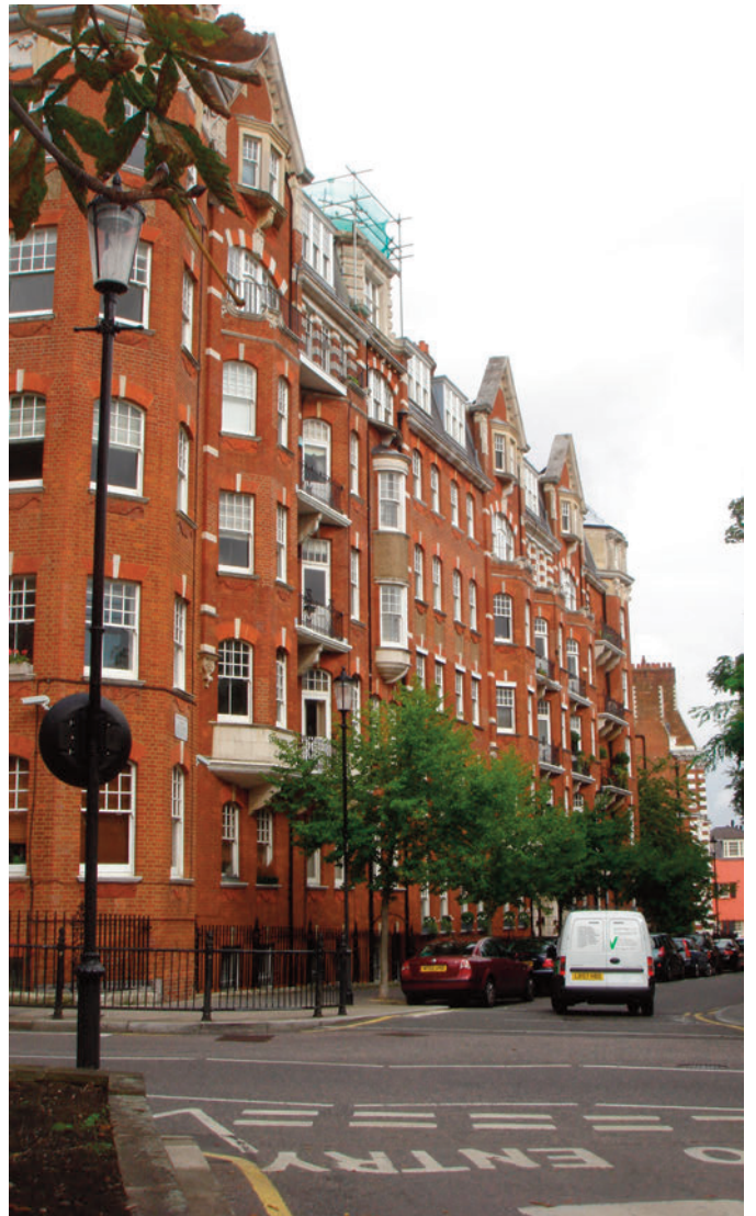
External repairs and decorations to a prestigious west London mansion block
