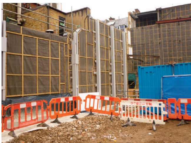
These 2 photographs show the site post-demolition with the temporary steels and weatherproofing fixed to the party wall.
