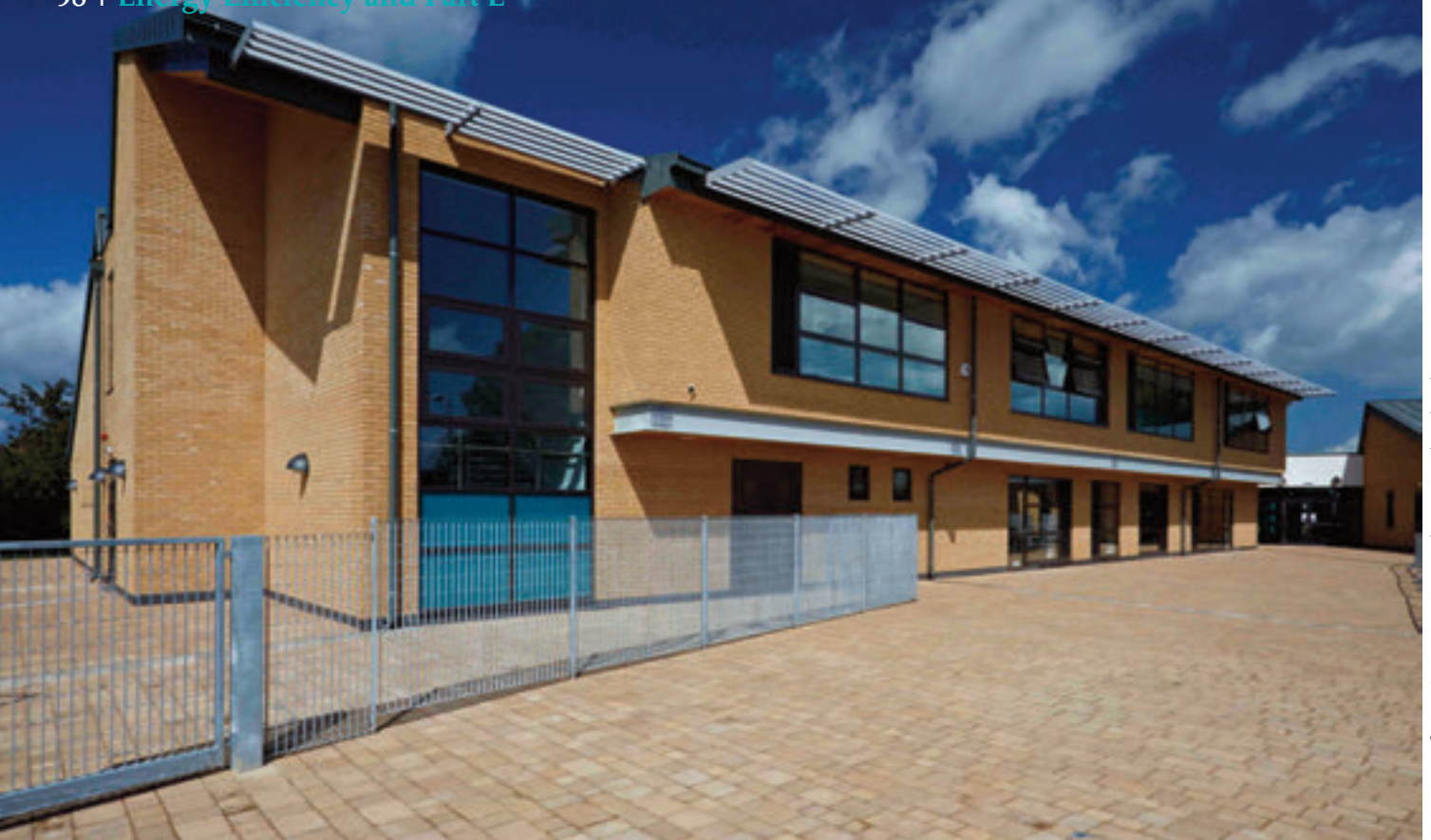
Courtesy of Kier Construction and Martin Cleveland
