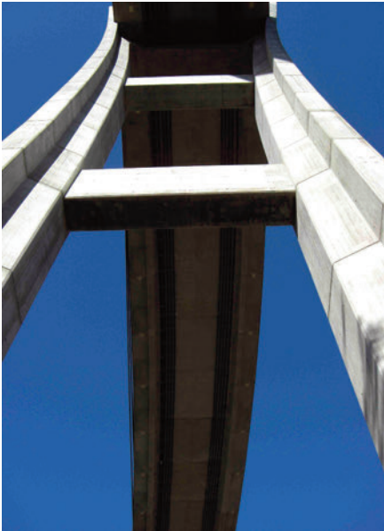
Figure 2: Some reinforced concrete structures are not easily accessible
