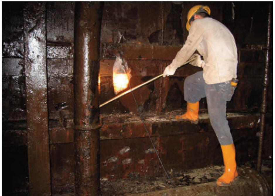
**CSR Primary function:** Rust and scale remover. Penetrates the substrate, expands during curing and separates the scale layers. Achieves pre-cleaning equivalent to ISO 8501-1, D Sa 2, or better.
