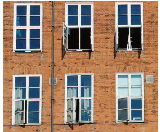
School facade in Copenhagen with window integrated heat recovery ventilation
