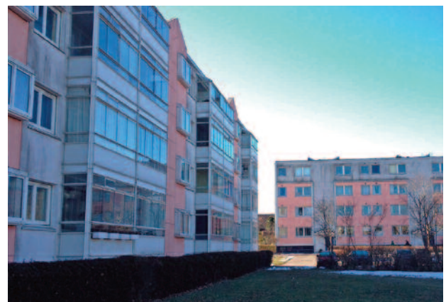
Ellebo today (before renovation)
