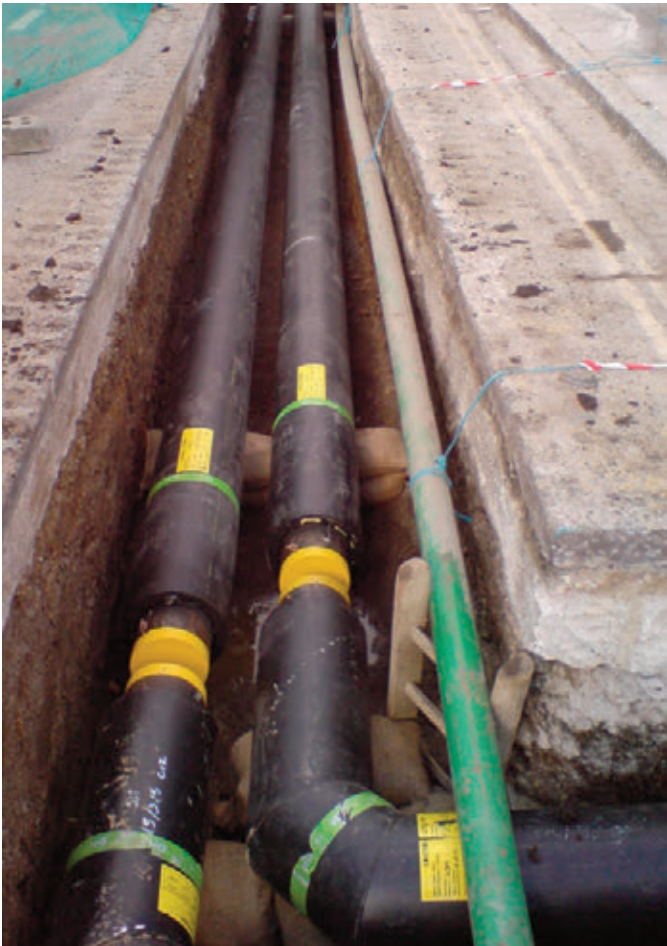
A relatively simple installation of district heating network in the highway. The pipes have been laid in place and are yet to be jointed
