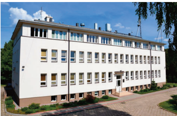
Administration and Laboratory building
