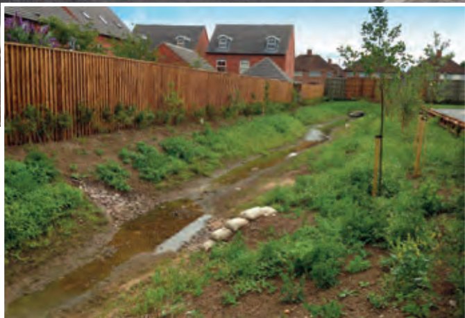
The Swale installation
