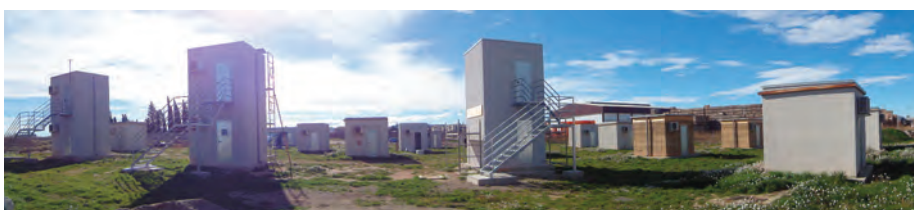
Pilot plant available at the University of Lleida, where TES is tested together with other energy efficiency technologies (good insulation, solar energy, heat pumps, etc.)
