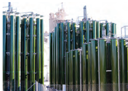
Figure 1. BFS' tested and certified (SGS) Industrial plant that absorbs CO 2 emitted from an adjacent cement factory.
