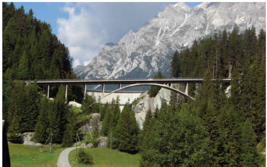
Figure 2: Typical highway bridge in the Swiss Mountains with severe exposure to de-icing salts in the winter
