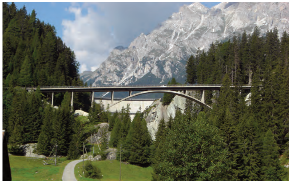
Figure 2: Typical highway bridge in the Swiss Mountains with severe exposure to de-icing salts in the winter
