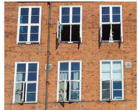
School facade in Copenhagen with window integrated heat recovery ventilation
