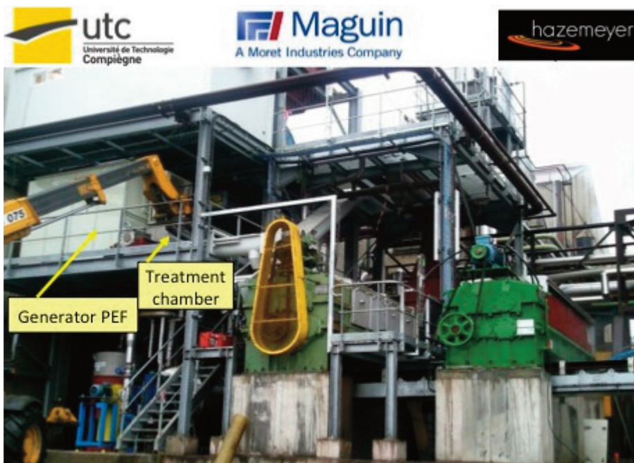
Figure 2: Industrial test of PEF (10t/hour) in sugar beet factory
