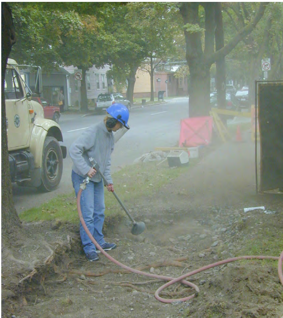
Using air excavation tools we uncover roots
