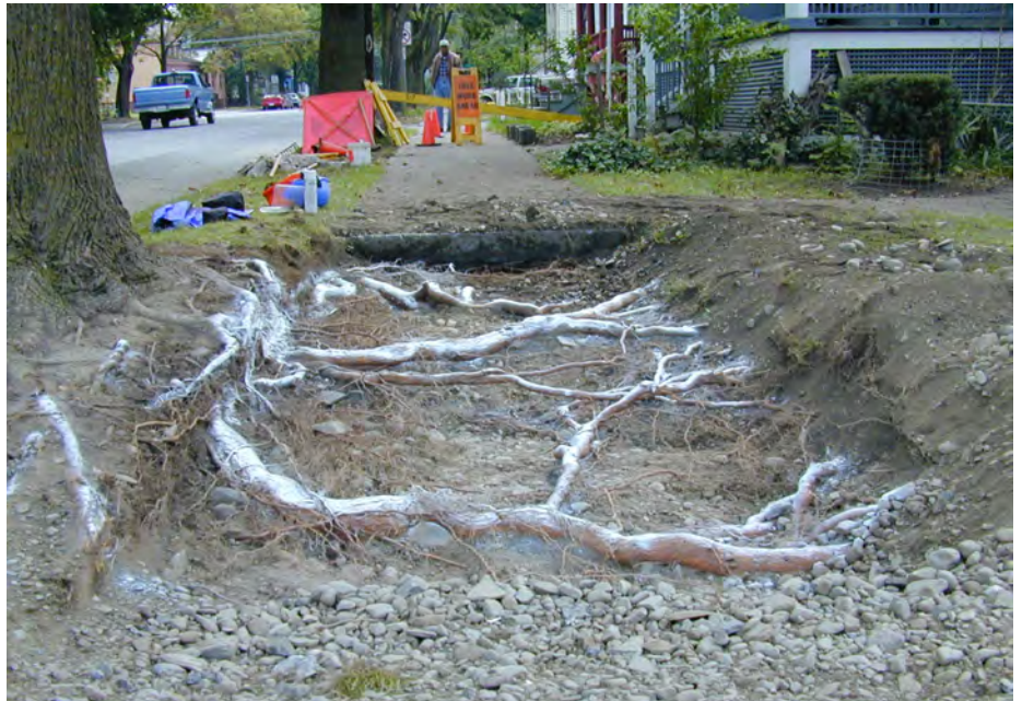
Tree roots escape a confined space by growing under a sidewalk into a neighbouring lawn
