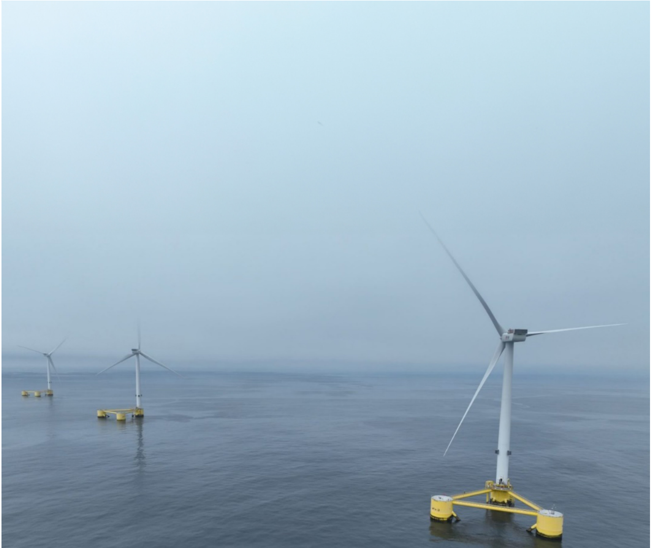
WindFloat Atlantic Project courtesy of Principle Power / Ocean Winds
