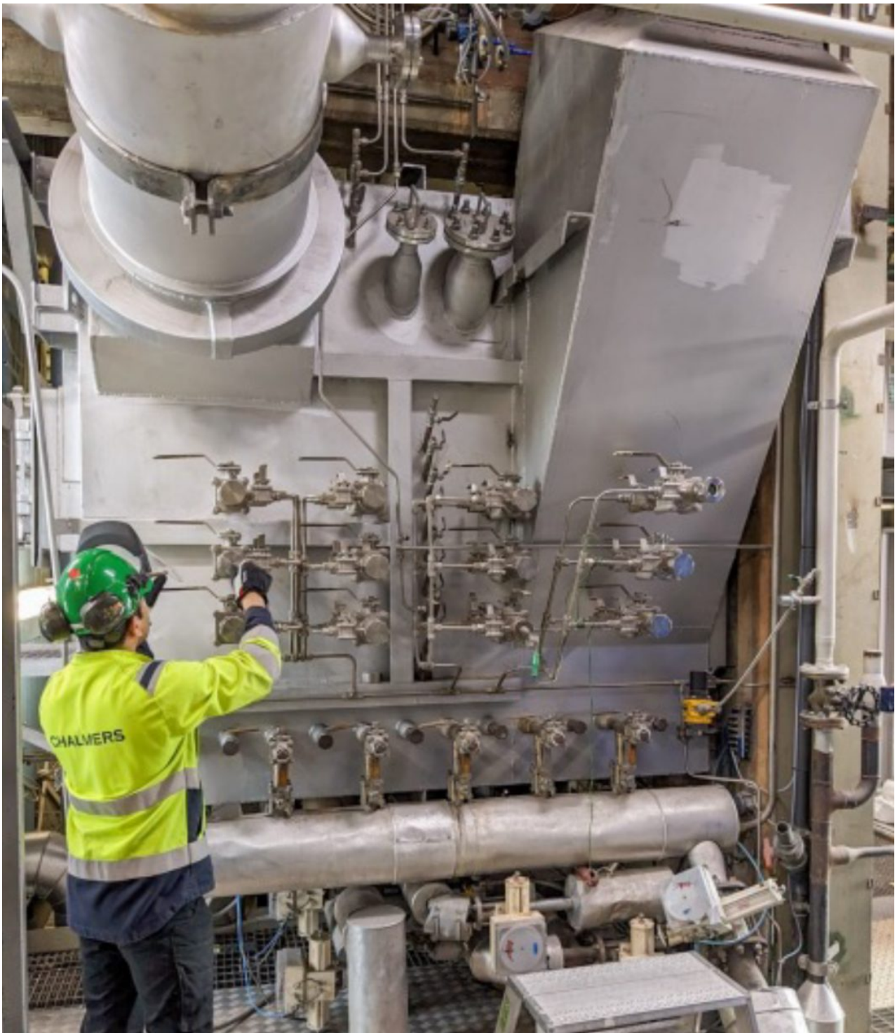
The 4-MWth Chalmers gasifier
