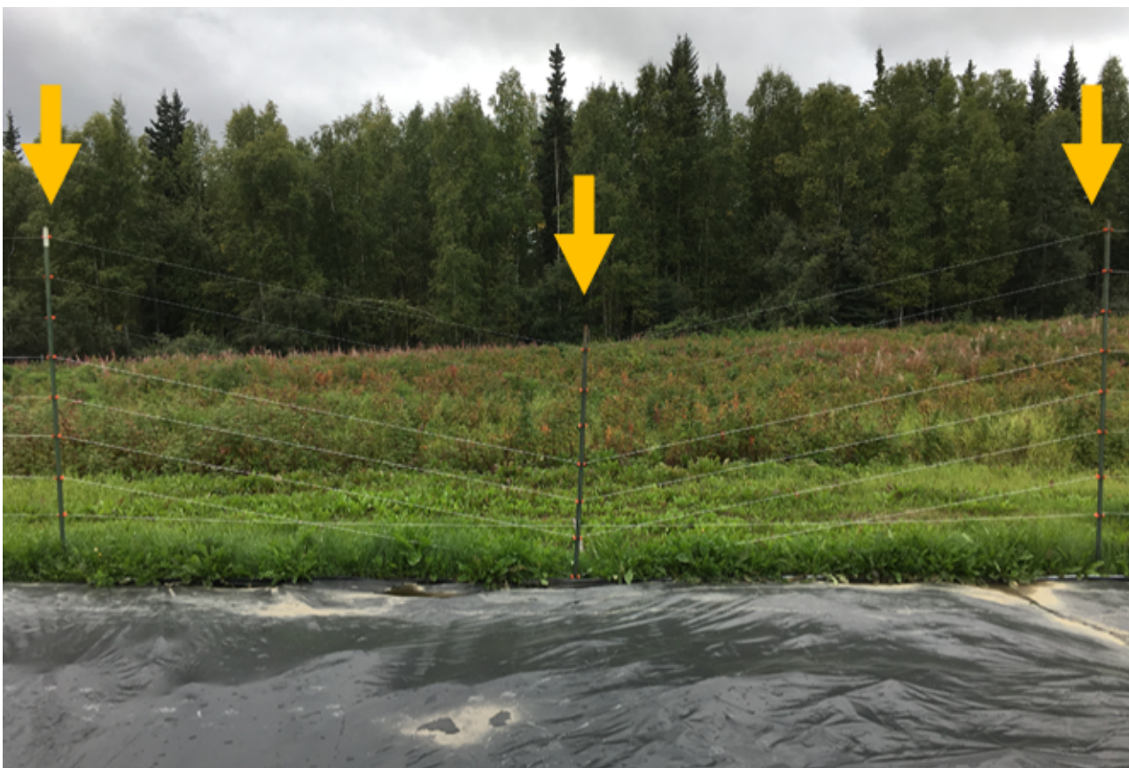
Figure 1: Black plastic mulch created a sinkhole and caused a fence post (marked by yellow arrows) to collapse during the 2019 growing season in Fairbanks, Alaska.
