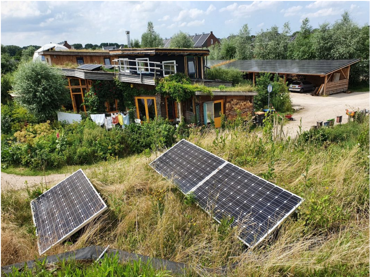
Figure: Aardehuizen house and EV-charging garage
